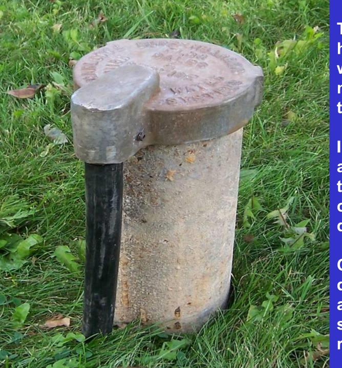
This drilled well has an older style well cap that does not seal tightly to the well casing.
