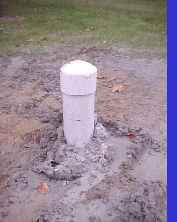
Temporary well cap - installed between well drilling and pump hook-up
